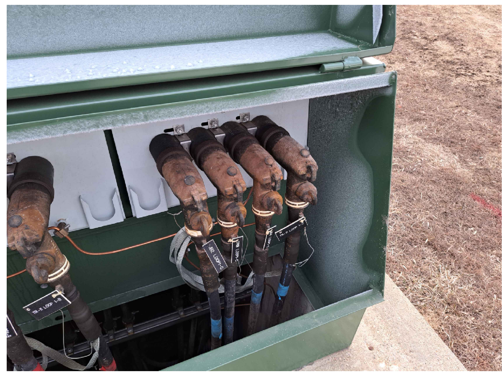
1 EXISTING CONDITIONS PHOTOS - 13,800 VOLTS - JBOX 3 NOT TO SCALE
