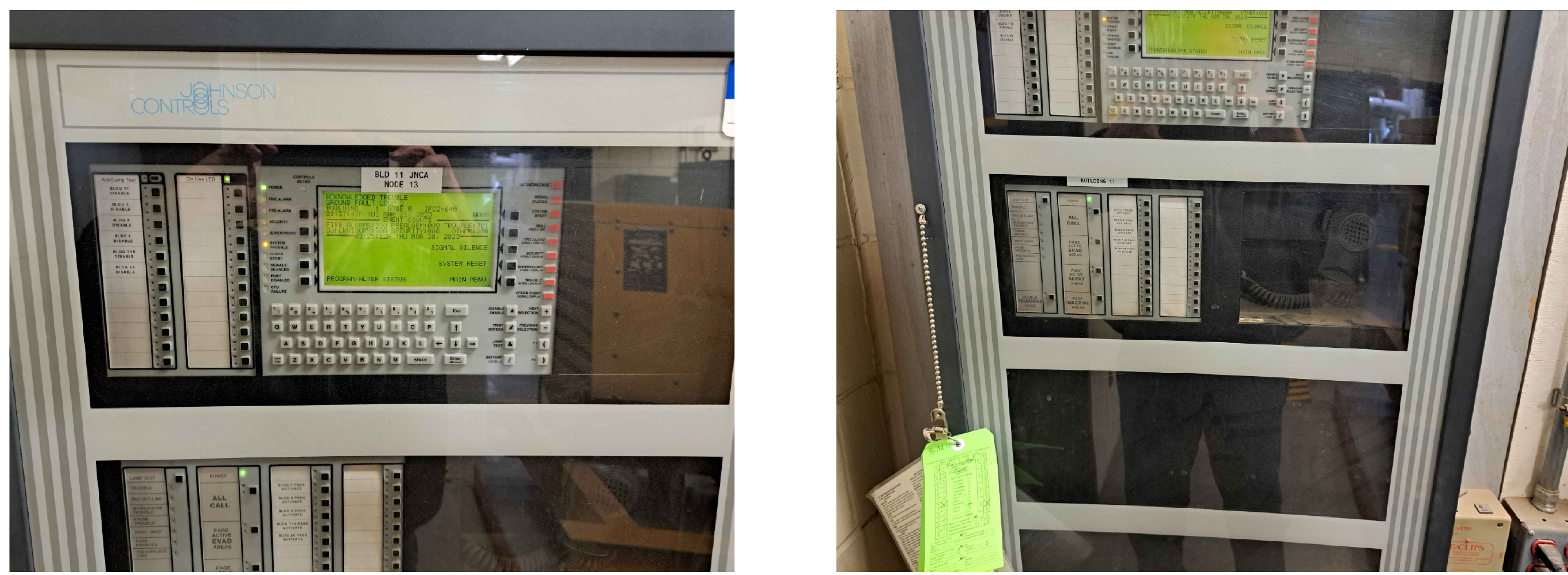
2 EXISTING FACP - BOILER BUILDING NOT TO SCALE
