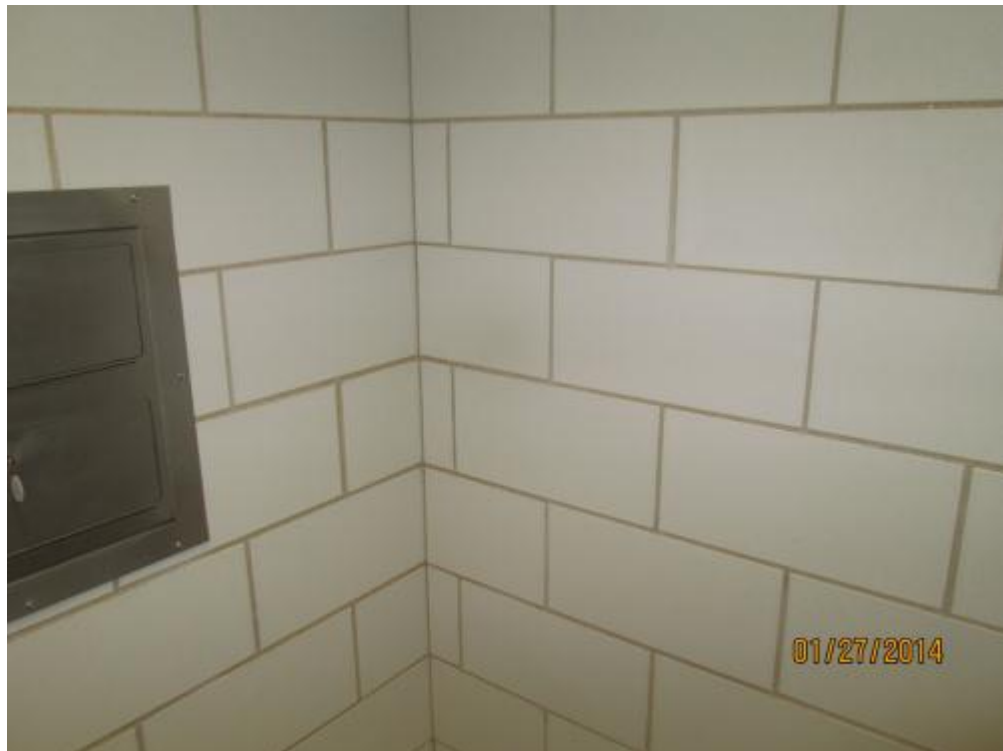
CTA02 – Ceramic Tile Adhesive – under 6"x12" white tile (Assumed).
