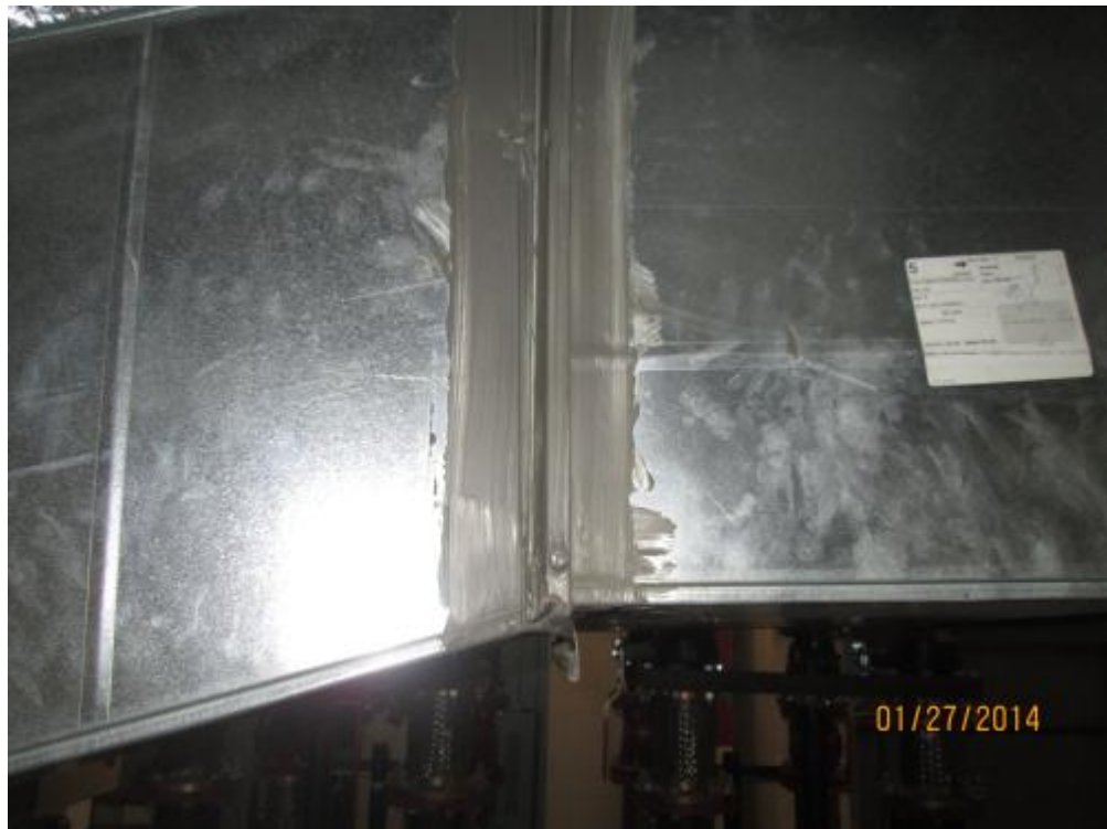
DTS01 – Duct Sealant – gray (No Asbestos Detected).
