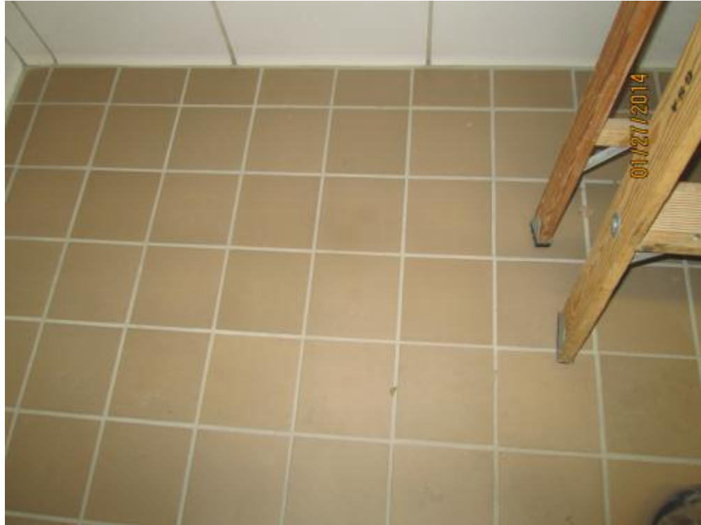
CTA01 – Ceramic Tile Adhesive – under 5"x5" tan tiles (Assumed).
