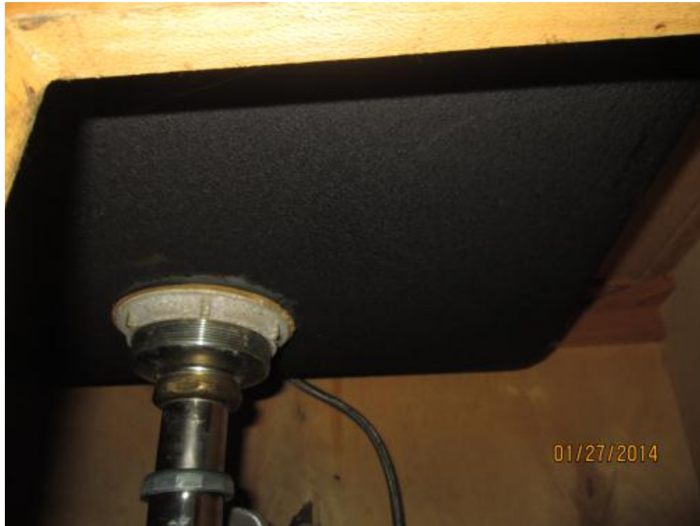
SUC02 – Sink Undercoating – black, rough (3% Chrysotile ).
