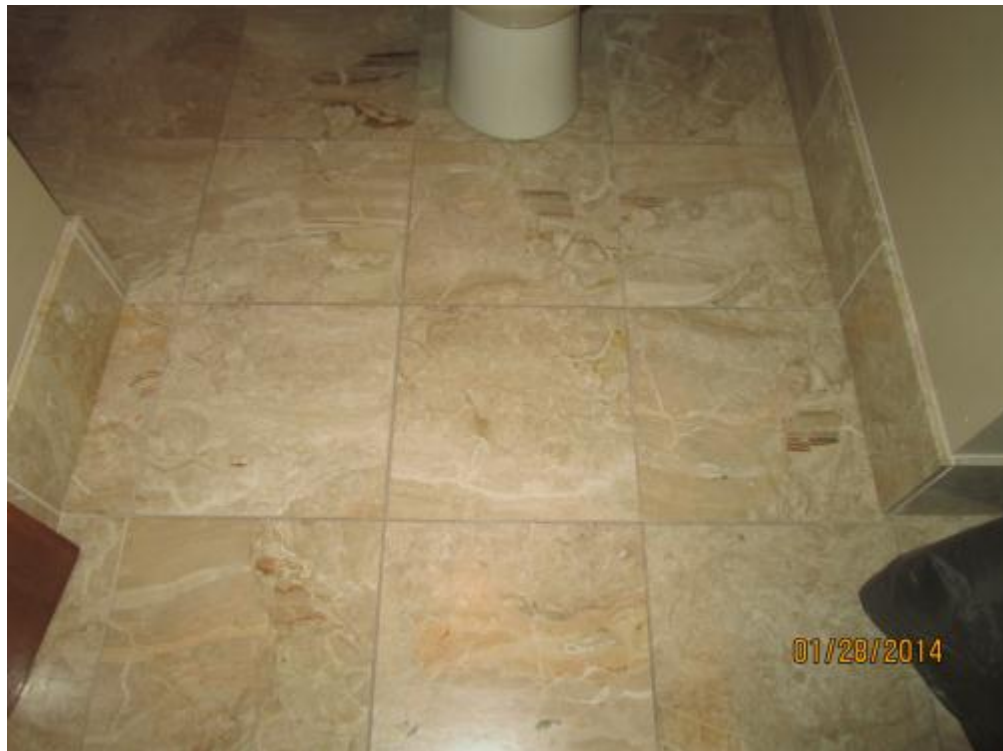
CTA04 – Ceramic Tile Adhesive – under tan marbled 12"x12" tile ( Assumed ).
