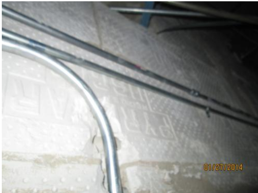
PL01 – Plaster – white plaster blocks (No Asbestos Detected).
