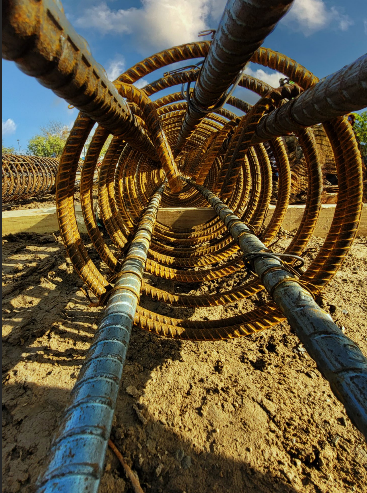
Figure 13: U.S. Courthouse Structure Greenville, MS
