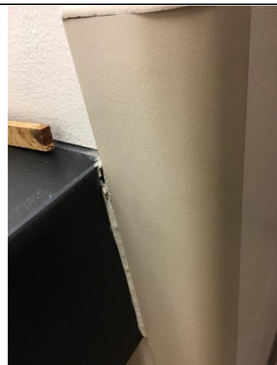
PHOTO 36 White Mastic – Lab Base Cabinets
