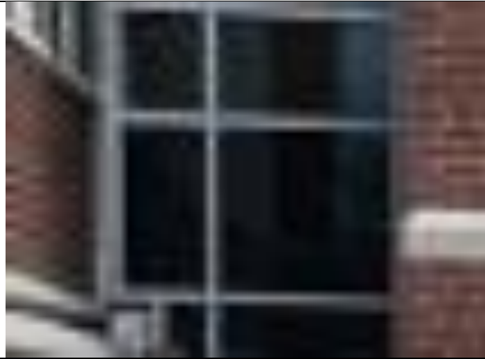
PHOTO 31 Silver Window Frame <1mg/cm 2 lead
