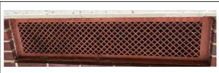
PHOTO 27 Red Ventilation Duct - Exterior <1mg/cm 2 lead
