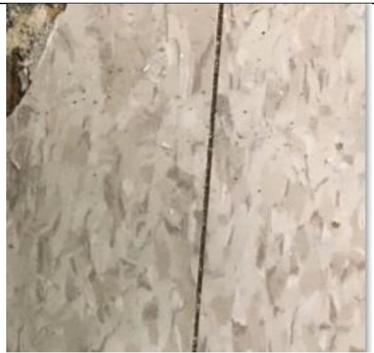
PHOTO 42 12" x 12" VFT Tan Blotchy/Mastic Black Mastic 4% Chrysotile
