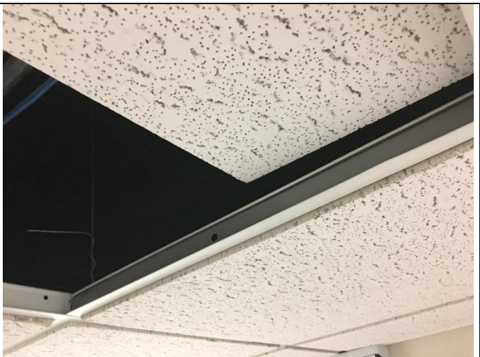
PHOTO 24 | 2' x 2' Ceiling Tile Hallway
