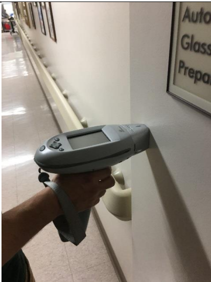
PHOTO 53 White Painted Wall – Hallway by D-17 <1mg/cm 2 lead
