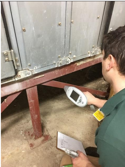
PHOTO 5 Red Painted Frame – Below Grade Mech. Room <1mg/cm 2 lead
