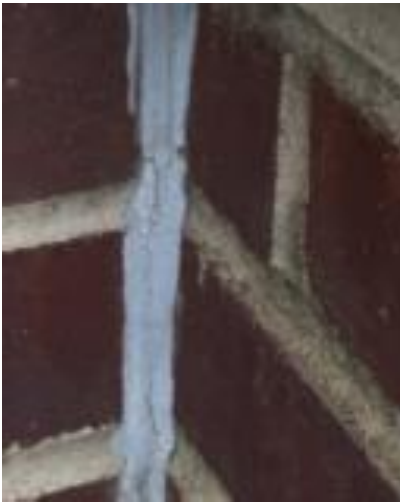
PHOTO 15 Gray Joint Caulk - Exterior
