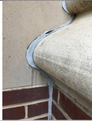
PHOTO 14 Gray Joint Caulk - Exterior
