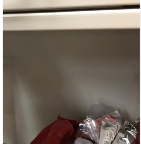
PHOTO 38 Plaster Wall – Lab (Exterior Wall)
