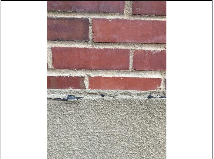
PHOTO 3 EFIS Surfacing – Mech. Room & Entry Area
