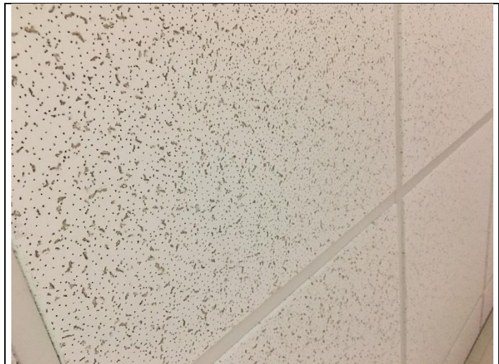
PHOTO 18 2' x 2' Ceiling Tile D-17
