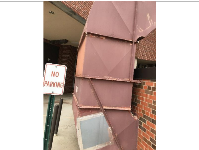
PHOTO 27 Red Ventilation Duct - Exterior <1mg/cm 2 lead
