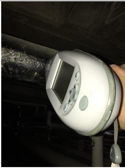
PHOTO 37 Black Pipe – Tunnel <1mg/cm 2 lead
