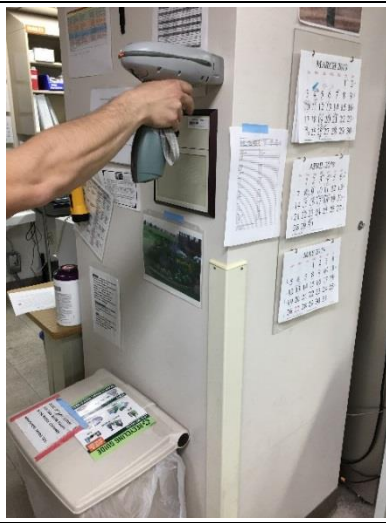
PHOTO 78 Plaster on column - Lab <1mg/cm 2 lead
