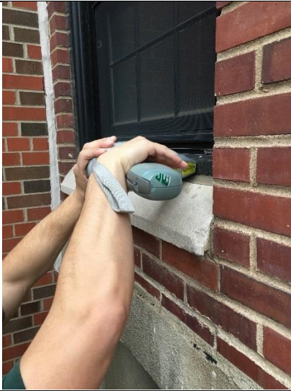
PHOTO 19 Black Window Frame - Exterior <1mg/cm 2 lead
