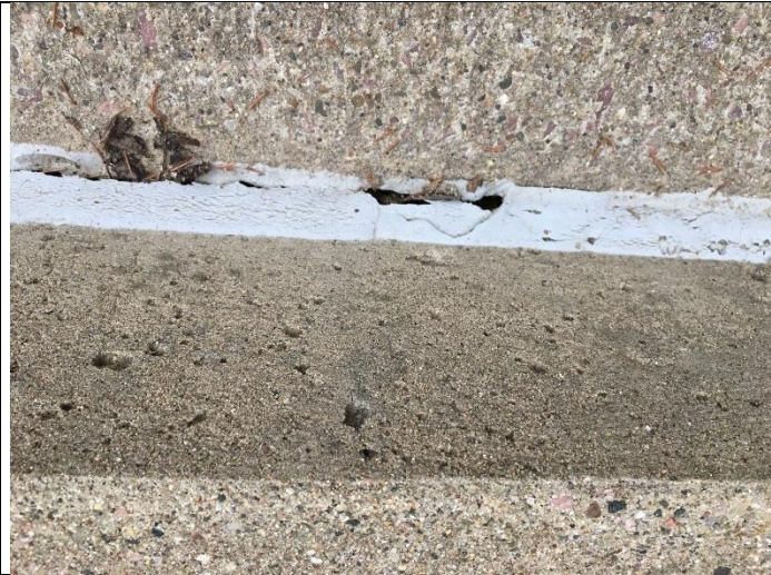
PHOTO 13 Gray Joint Caulk – Horizontal Concrete Pad
