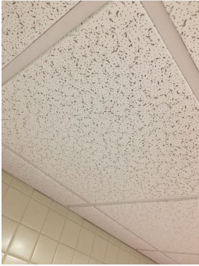
PHOTO 19 | 2' x 2' Ceiling Tile D-17
