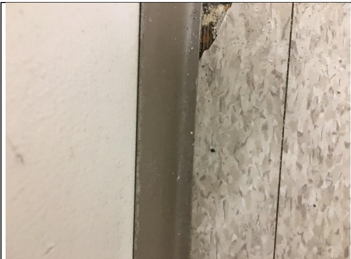
PHOTO 41 12" x 12" VFT Tan Blotchy/Mastic Black Mastic 4% Chrysotile
