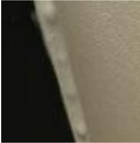
PHOTO 37 White Mastic – Lab Base Cabinets
