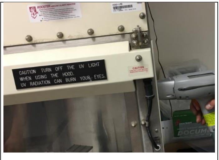
PHOTO 70 Cream Fume Hood – West Wall <1mg/cm 2 lead
