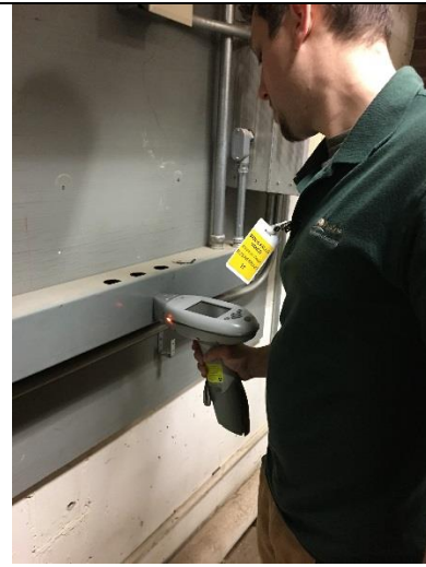
PHOTO 10 Gray Painted Casing – Below Grade Mechanical Room <1mg/cm 2 lead
