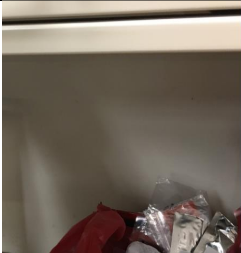
PHOTO 39 Plaster Wall – Lab (Exterior Wall)
