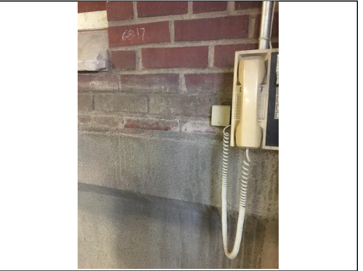
PHOTO 4 EFIS Surfacing – Mech. Room & Entry Area
