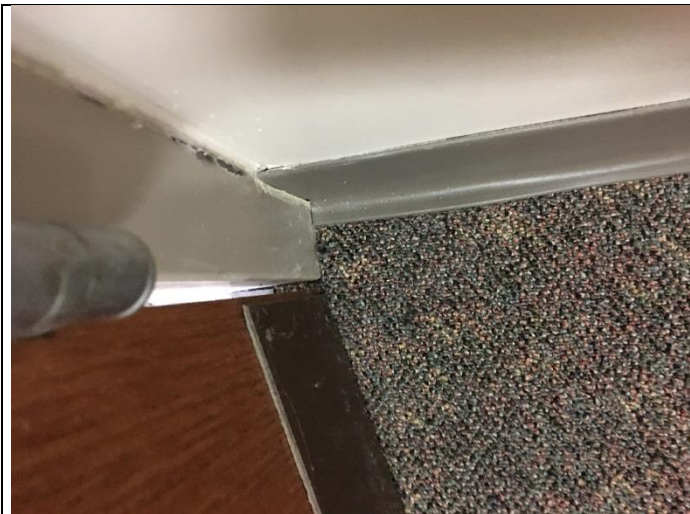
PHOTO 47 12" x 12" VFT Tan/Black Mastic Under Carpet D-22
