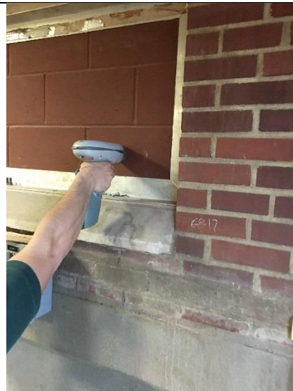
PHOTO 6 Red Painted Block Wall – Below Grade Mech. Rm <1mg/cm 2 lead
