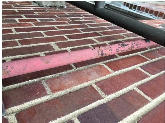
PHOTO 25 Red Pipe - Exterior <1mg/cm 2 lead
