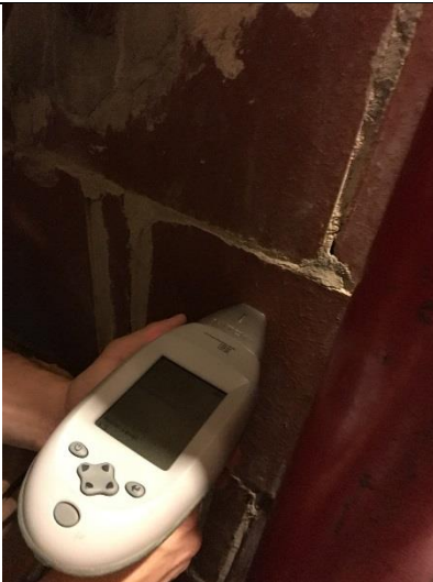
PHOTO 45 Metal Door Frame to East Stairwell Tower 3 <1mg/cm 2 lead
