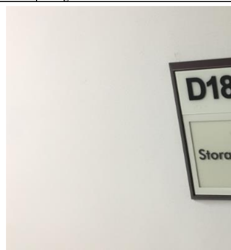
PHOTO 60 Cream Painted Sheetrock Wall - Hallway <1mg/cm 2 lead
