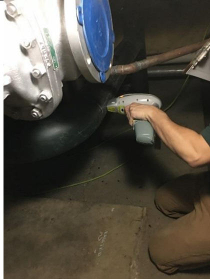
PHOTO 38 Black Pipe – Tunnel <1mg/cm 2 lead
