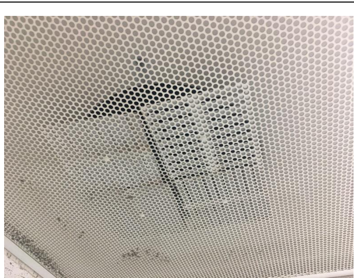
PHOTO 54 Diffuser Grate – Hallway by D-17 <1mg/cm 2 lead
