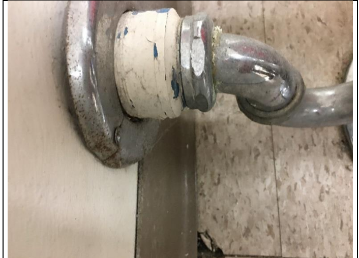
PHOTO 40 12" x 12" VFT Tan Blotchy/Mastic Black Mastic 4% Chrysotile
