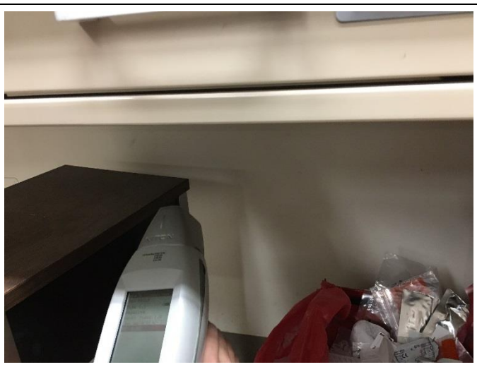
PHOTO 76 White Paint on Plaster <1mg/cm 2 lead
