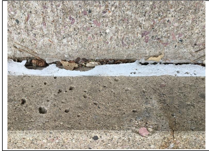
PHOTO 12 | Gray Joint Caulk – Horizontal Concrete Pad
