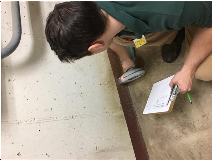
PHOTO 3 Red Base Cove Paint – Below Grade Mech. Room <1mg/cm 2 lead
