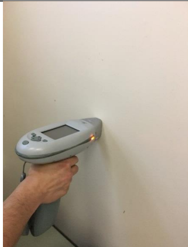
PHOTO 82 North Wall - D-20 <1mg/cm 2 lead
