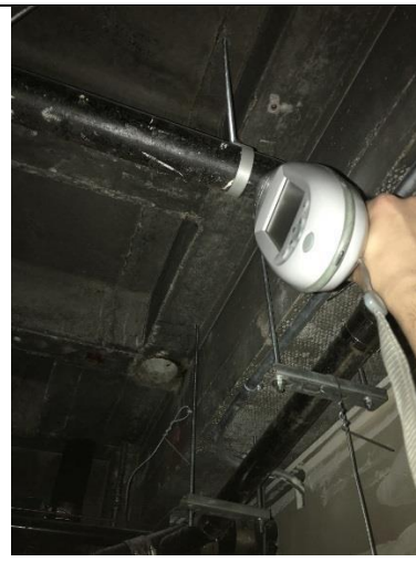
PHOTO 52 Black Pipe D-17 Hallway <1mg/cm 2 lead
