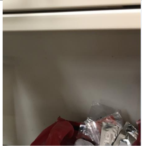
PHOTO 38 Plaster Wall – Lab (Exterior Wall)
