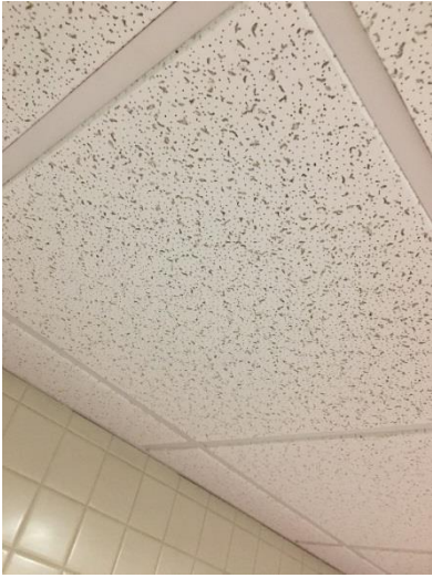
PHOTO 19 | 2' x 2' Ceiling Tile D-17
