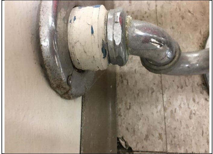
PHOTO 40 12" x 12" VFT Tan Blotchy/Mastic Black Mastic 4% Chrysotile
