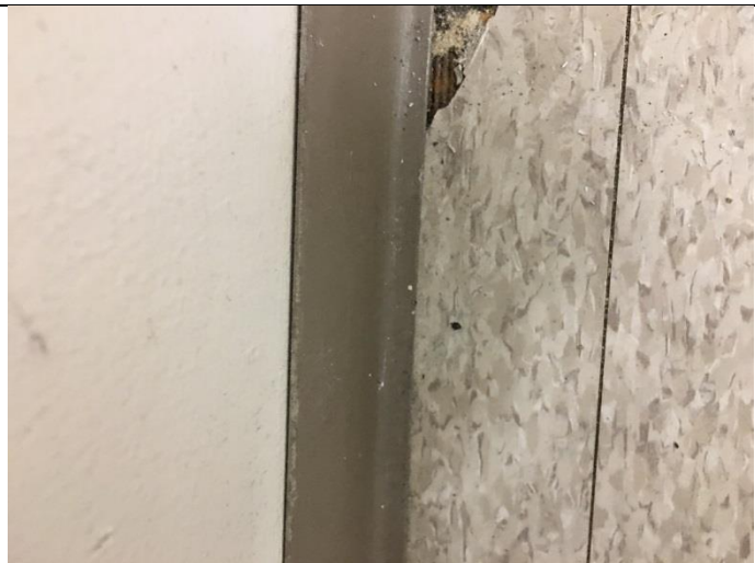
PHOTO 41 12" x 12" VFT Tan Blotchy/Mastic Black Mastic 4% Chrysotile
