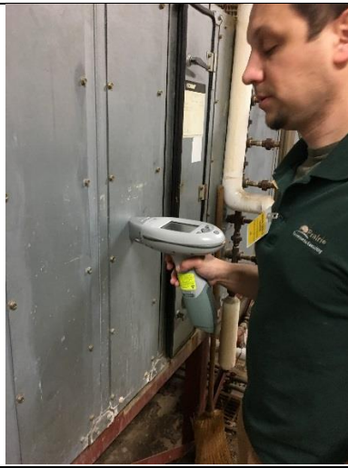
PHOTO 4 Electrical Panel – Below Grade Mechanical Room <1mg/cm 2 lead
