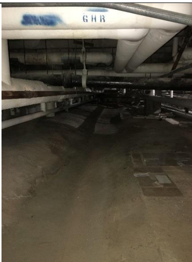
PHOTO 34 Black Pipe – Tunnel <1mg/cm 2 lead
