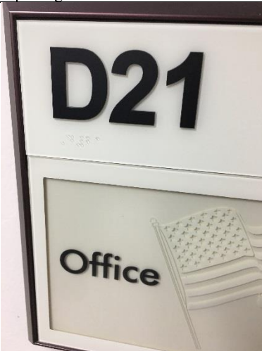
PHOTO 59 Cream Painted Sheetrock Wall – Room D-21 <1mg/cm 2 lead
