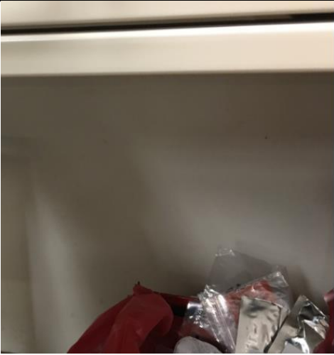
PHOTO 39 Plaster Wall – Lab (Exterior Wall)
