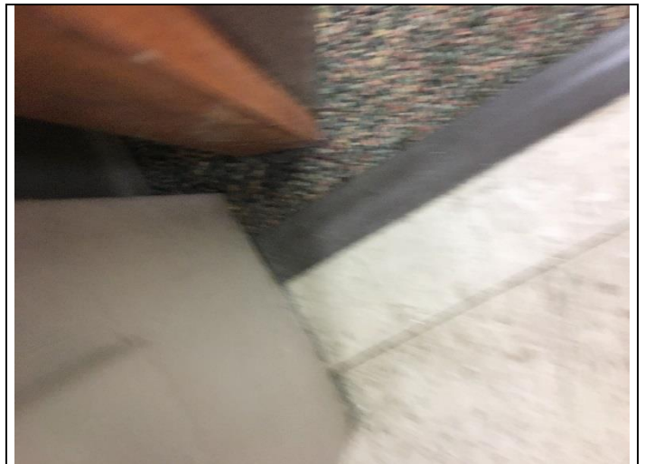
PHOTO 48 12" x 12" VFT Tan/Black Mastic Under Carpet D-22
