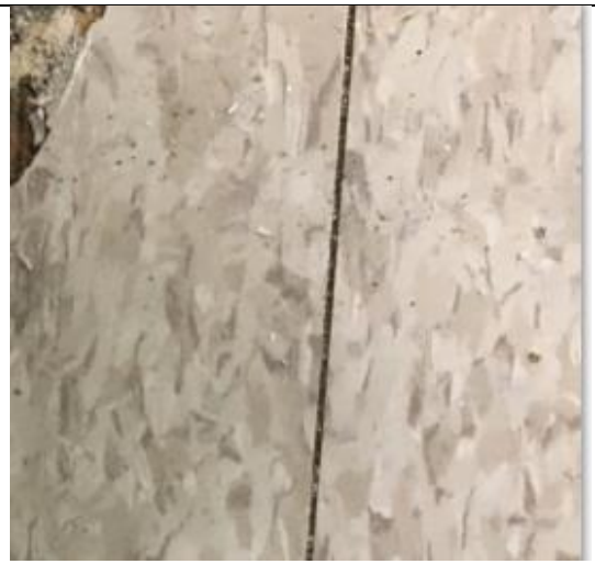
PHOTO 42 12" x 12" VFT Tan Blotchy/Mastic Black Mastic 4% Chrysotile
