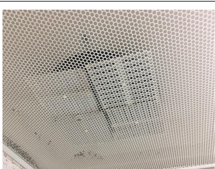
PHOTO 54 Diffuser Grate – Hallway by D-17 <1mg/cm 2 lead
