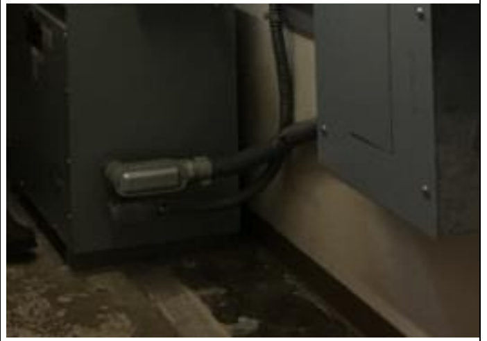
PHOTO 44 Black Mastic – D-20 5% Chrysotile
