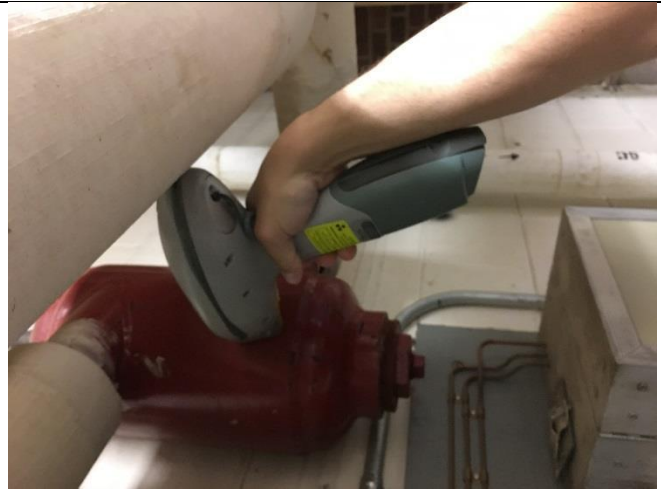
PHOTO 8 Red Painted Mixing Chamber – Below Grade Mech. Room <math><1\text{mg}/\text{cm}^2</math> lead
