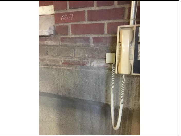
PHOTO 4 | EFIS Surfacing – Mech. Room & Entry Area
