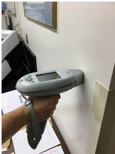
PHOTO 73 White Painted Sheetrock Wall - Lab <1mg/cm 2 lead
