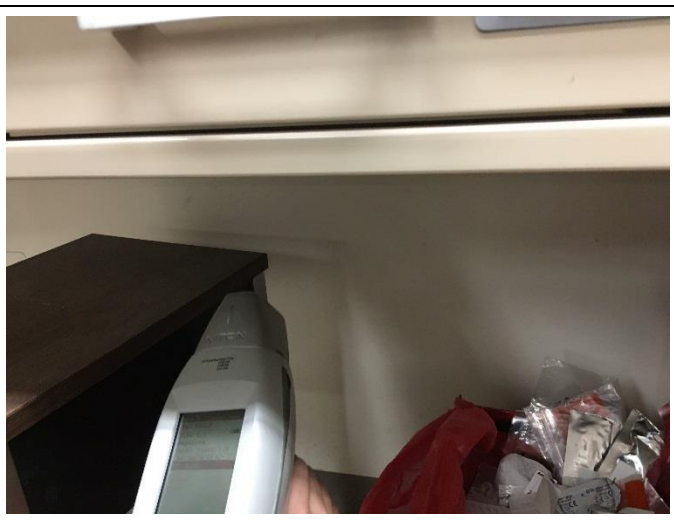
PHOTO 76 White Paint on Plaster <1mg/cm 2 lead
