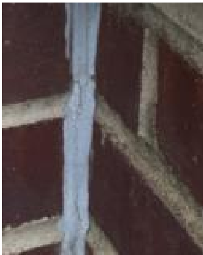
PHOTO 15 Gray Joint Caulk - Exterior
