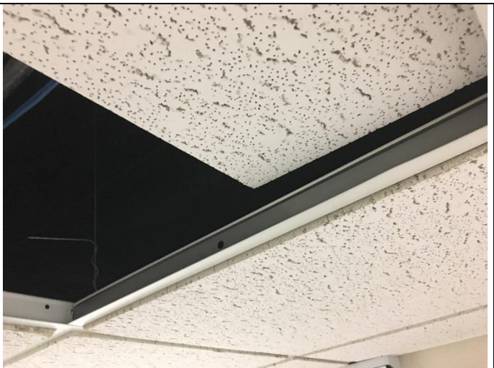
PHOTO 24 | 2' x 2' Ceiling Tile Hallway
