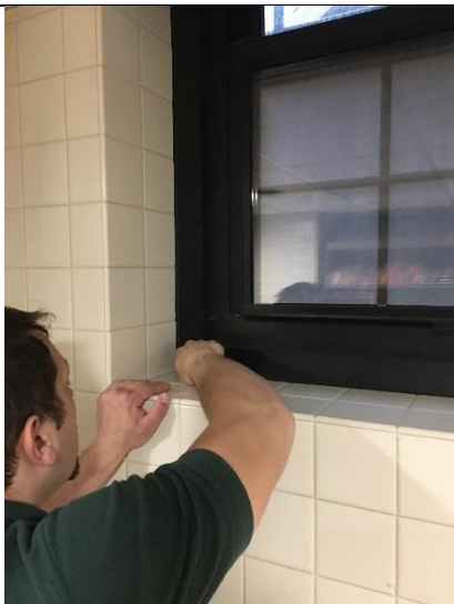
PHOTO 23 | Black Window Caulk – Windows Throughout
