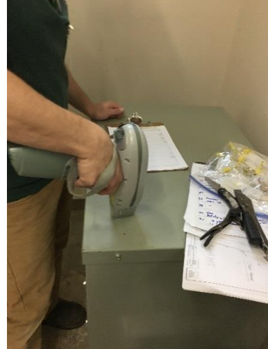
PHOTO 80 Transformer Box - D -20 <1mg/cm 2 lead
