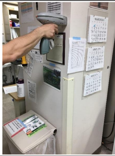
PHOTO 78 Plaster on column - Lab <1mg/cm 2 lead
