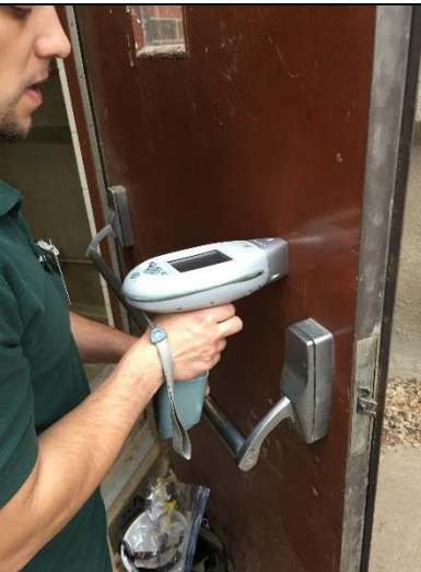
PHOTO 21 Red Mech. Room Door (Inside) <1mg/cm 2 lead
