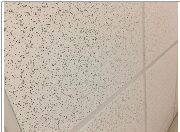
PHOTO 18 2' x 2' Ceiling Tile D-17
