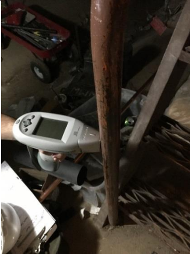
PHOTO 39 Brown Hand Railing-Stairs to Tunnel 3.8 mg/cm 2 lead
