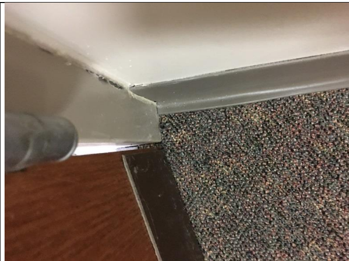
PHOTO 47 12" x 12" VFT Tan/Black Mastic Under Carpet D-22
