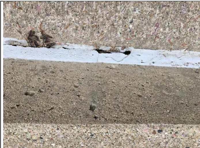
PHOTO 13 Gray Joint Caulk – Horizontal Concrete Pad
