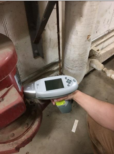
PHOTO 11 Red Painted Mixing Chamber – Below Grade Mech. Room <math><1\text{mg}/\text{cm}^2</math> lead
