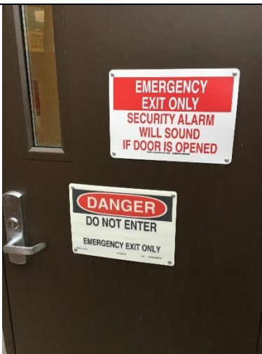
PHOTO 23 Brown Door (Outside) <1mg/cm 2 lead
