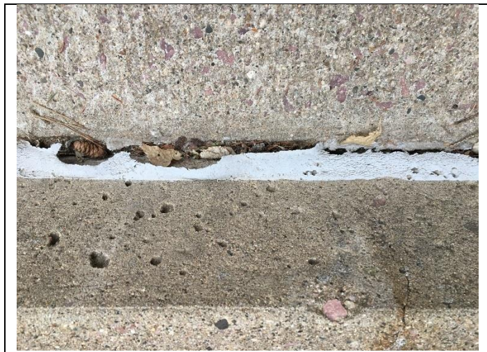
PHOTO 12 Gray Joint Caulk – Horizontal Concrete Pad
