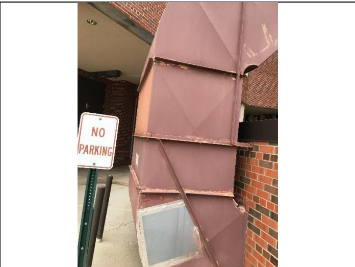
PHOTO 27 Red Ventilation Duct - Exterior <1mg/cm 2 lead
