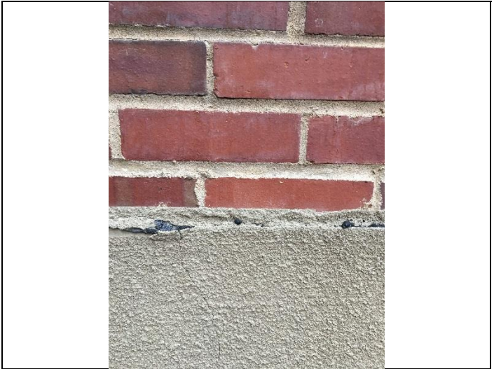
PHOTO 3 | EFIS Surfacing – Mech. Room & Entry Area
