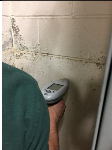
PHOTO 2 White Painted wall - Below Grade Mech. Room <1mg/cm 2 lead
