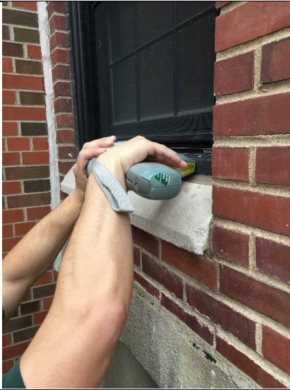
PHOTO 19 Black Window Frame - Exterior <1mg/cm 2 lead
