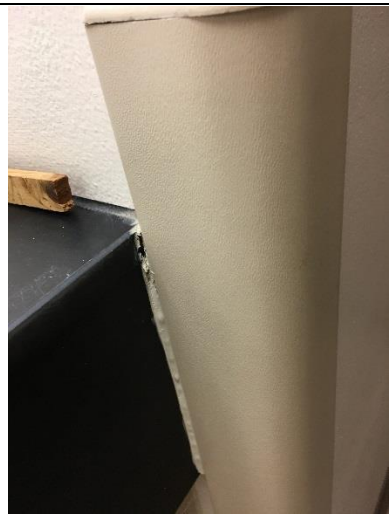
PHOTO 36 White Mastic – Lab Base Cabinets
