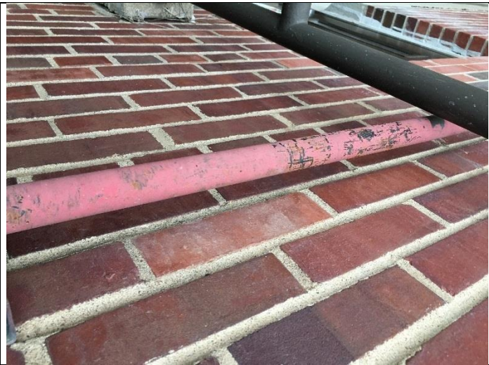
PHOTO 25 Red Pipe - Exterior <1mg/cm 2 lead
