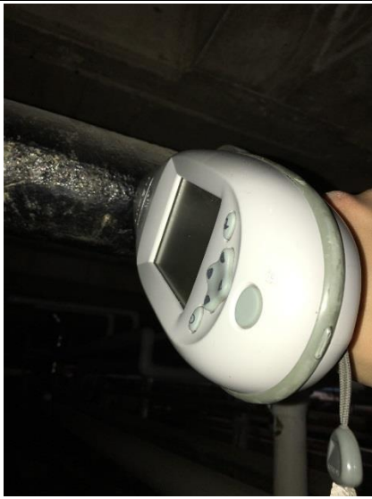
PHOTO 37 Black Pipe – Tunnel <1mg/cm 2 lead
