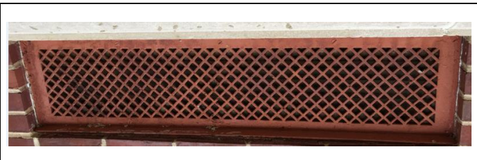
PHOTO 27 Red Ventilation Duct - Exterior <1mg/cm 2 lead
