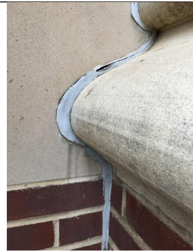
PHOTO 14 Gray Joint Caulk - Exterior
