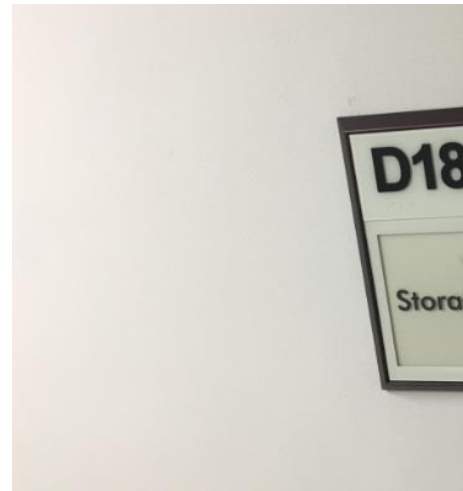
PHOTO 60 Cream Painted Sheetrock Wall - Hallway <1mg/cm 2 lead
