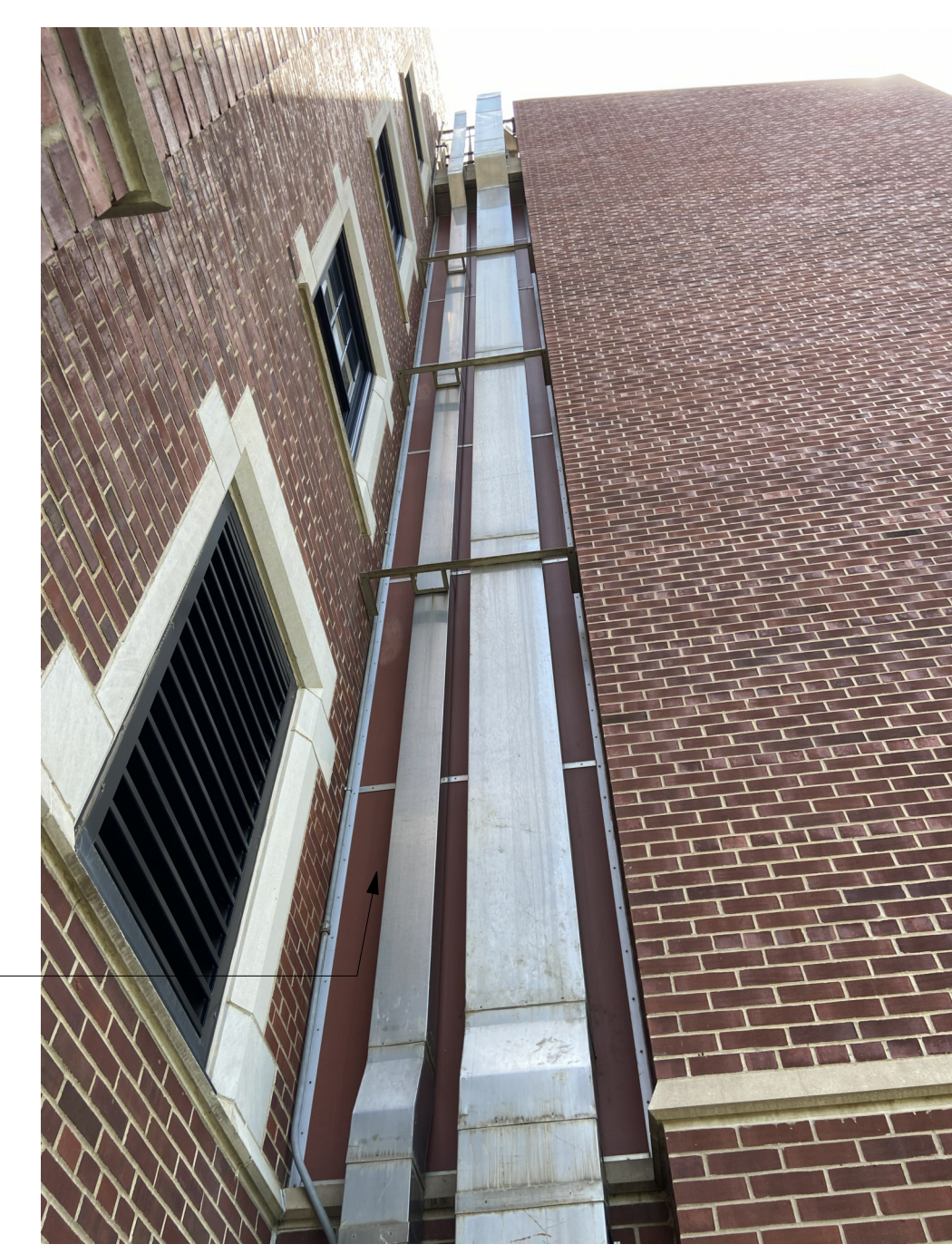
EXISTING CONDITIONS - DUCTWORK & SUPPORTS AND PANELING ON EXTERIOR
